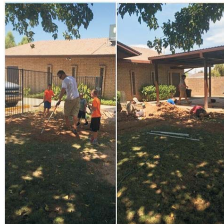
Working on Sprinklers
