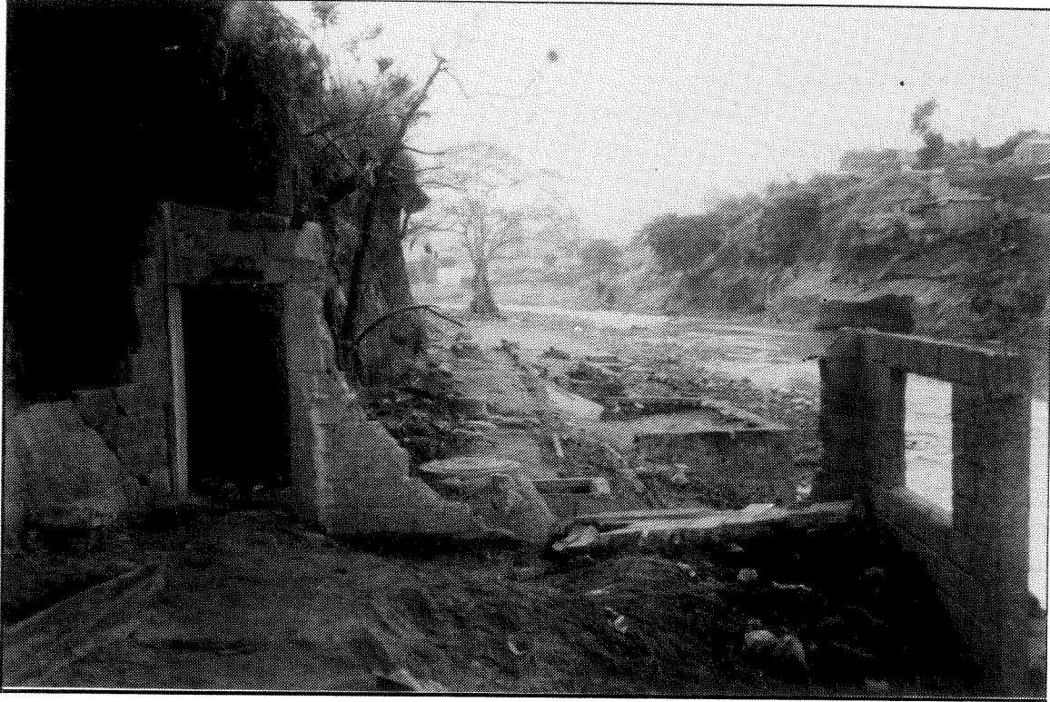
▶ TEGUCIGALPA—THIS WAS A HOUSING PROJECT.
