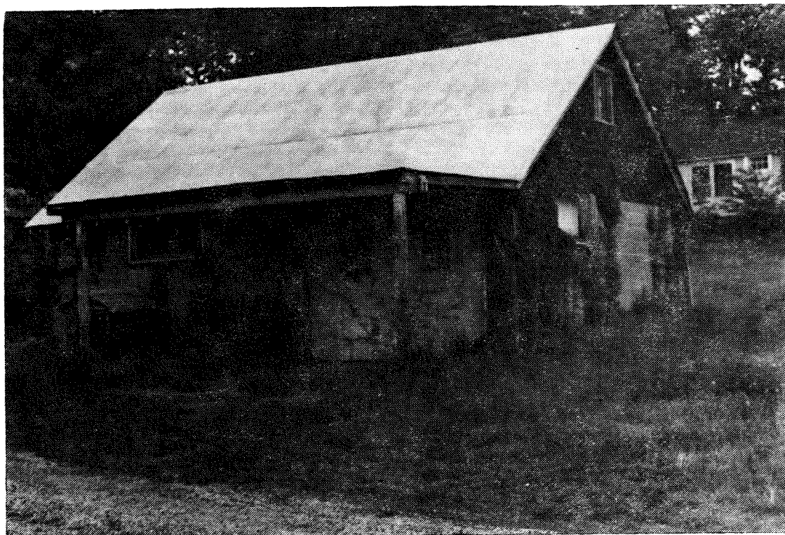
SISTER ORA DERRY'S GARAGE
